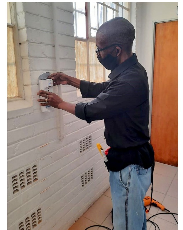
// Installation of Automatic Hand Sanitisers
